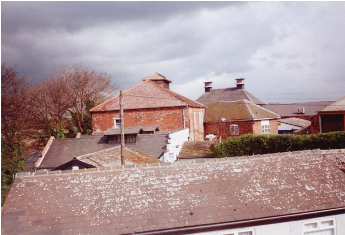
Plate 9 : Former Brewery Buildings, off London Road
