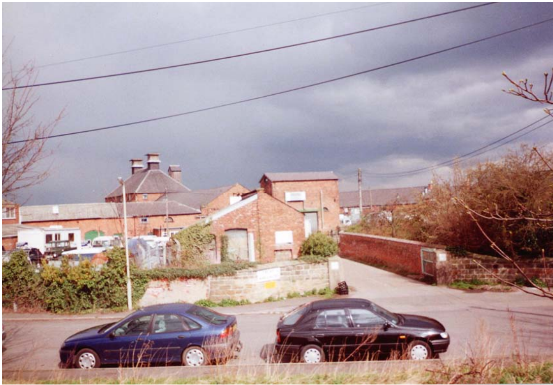
Plate 8 : Former Brewery Buildings, off London Road
