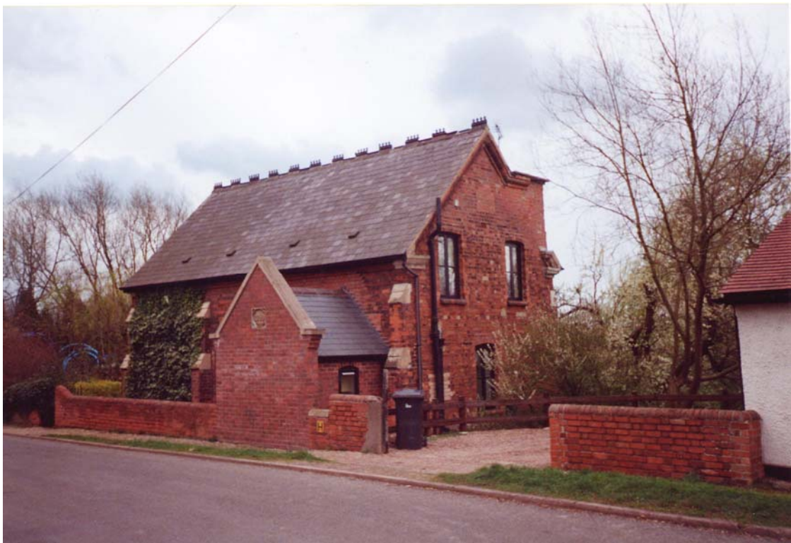
Plate 3 : Former School (now Cavendish House)
