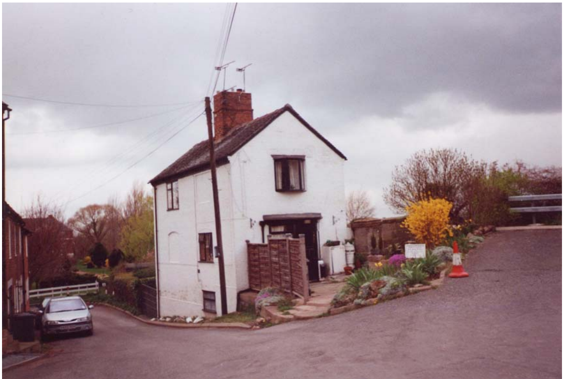
Plate 18 : Whitewash Facades to No. 11 Cavendish Bridge
