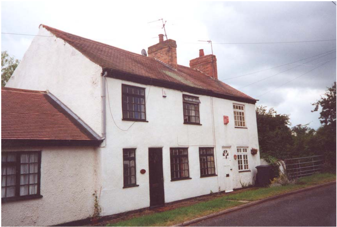
Plate 17 : Modern Window Units and Whitewashed Facades to 'Homelea'
