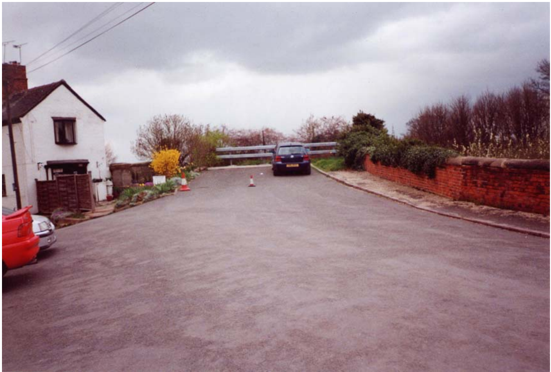
Plate 10 : Boundary Walls at Approach to former Cavendish Bridge
