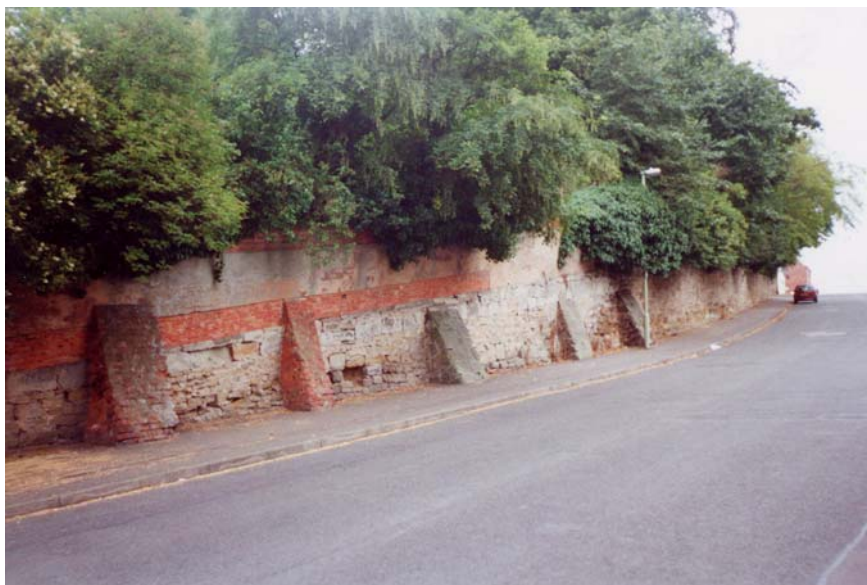
Plate 35 Wall to (former) Vicarage Grounds, Delven Lane
