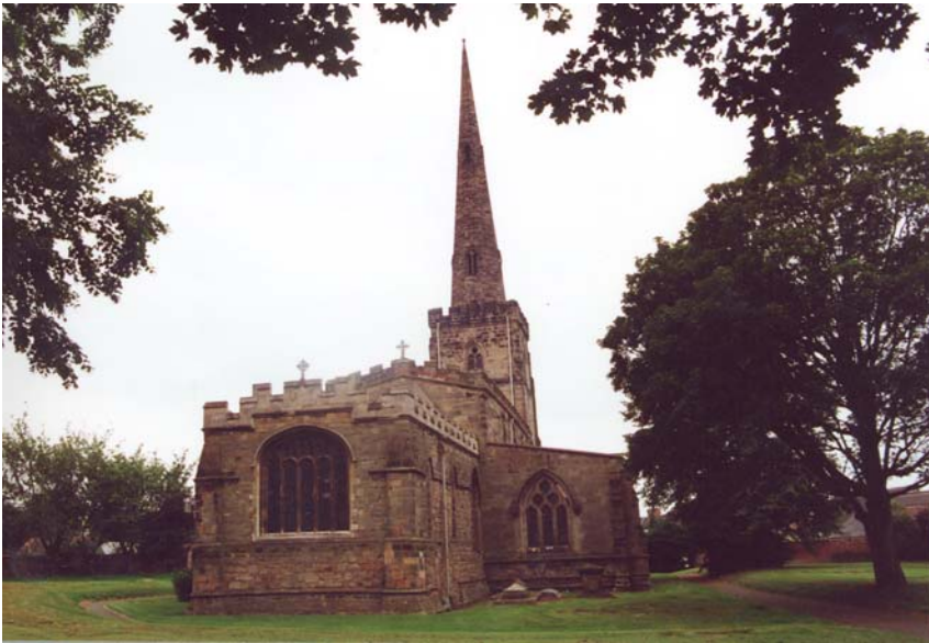
Plate 5 Parish Church of St. Edward, King And Martyr, Clapgun Street
