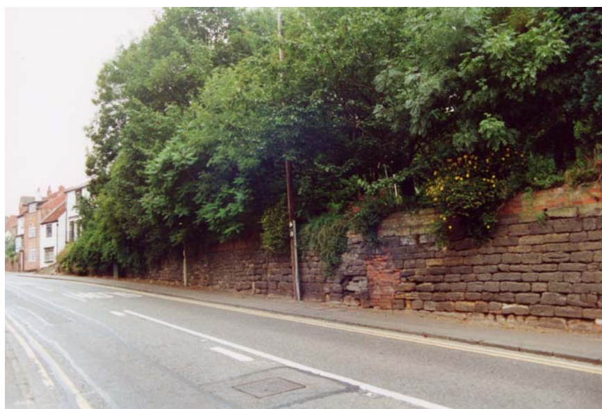
Plate 36 Retaining Walls on the Western side of Bondgate
