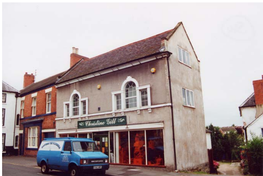
Plate 54 Nos. 3/5 Borough Street : PvcU Window Units at First Floor Level
