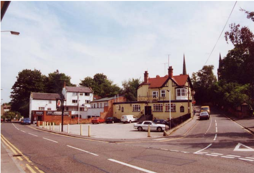
Plate 47 Car Parking Area to Turks Head Public House, Bondgate/Market Street
