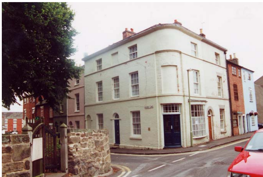
Plate 22 Properties to the North- Eastern side of Church Lane
