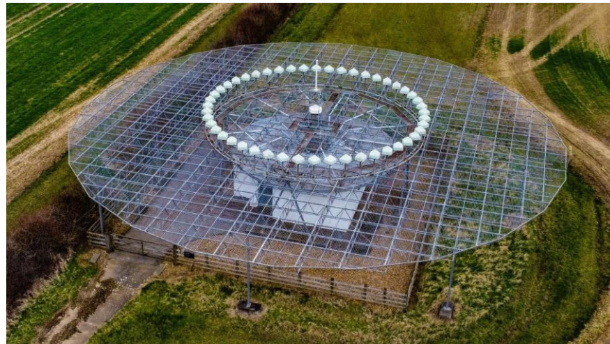
The Daventry Doppler VHF Omni-directional Range (MCT DVOR). A ground-based radio navigation beacon used by pilots to assist in aircraft navigation.
