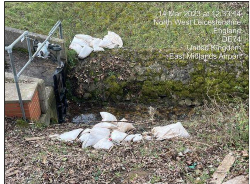
Photograph 4: Site A Hotel Upstream.
